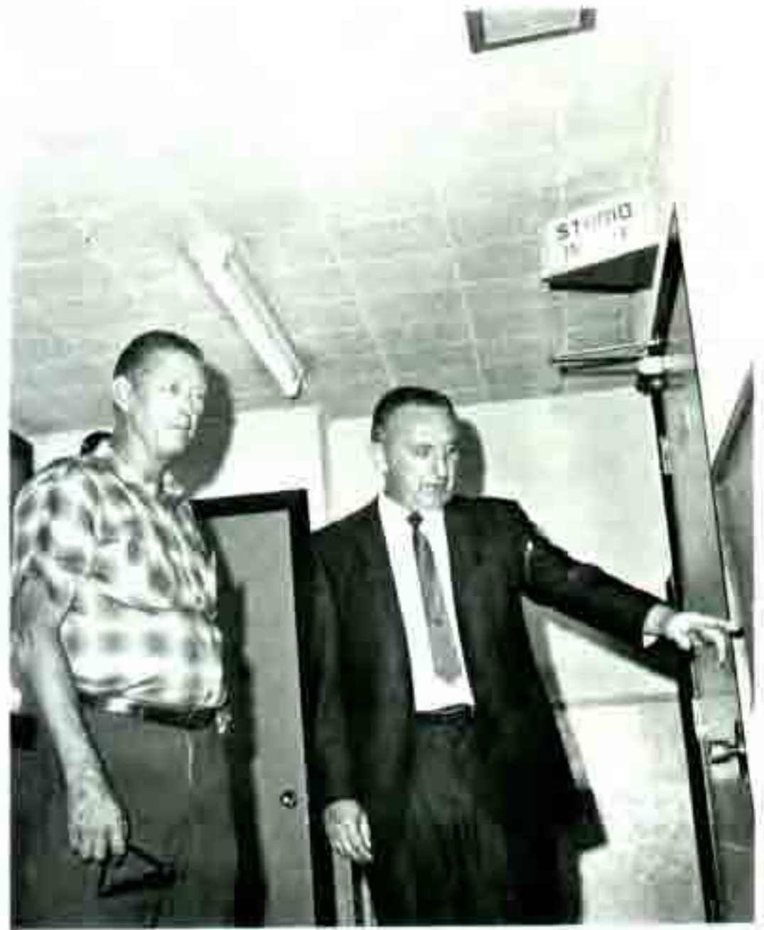
Renovation of studios included complete resurfacing of main corridor walls.
