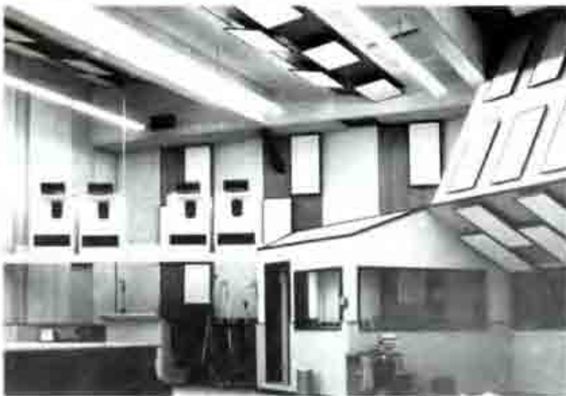
The recent up-dating of United's busy Studio A included construction of a fully enclosed vocal booth for separation of solo instrumental or vocal parts.
